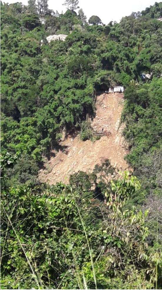
Figure 6. Landslide L3 . This landslide occurred in a series of interbedded sandstones and shales of the Wag Water Formation. This is an area of folding and the sandstones and shales are dipping downslope towards the road (which is situated at the foot of the landslide). Photograph by SFM .
